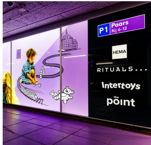
Cityplaza & Winkelhof: Switching to >800 LEDs in the parking garages saves 50% energy
