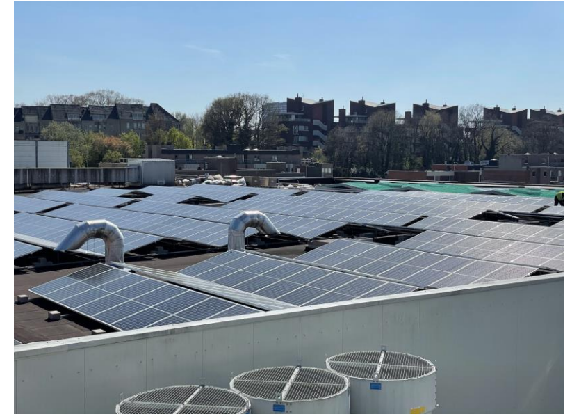
Shopping 1 Genk: 1.765 solar panels installed, 450 kWp capacity. This is about 20% of the shared services electricity consumption
