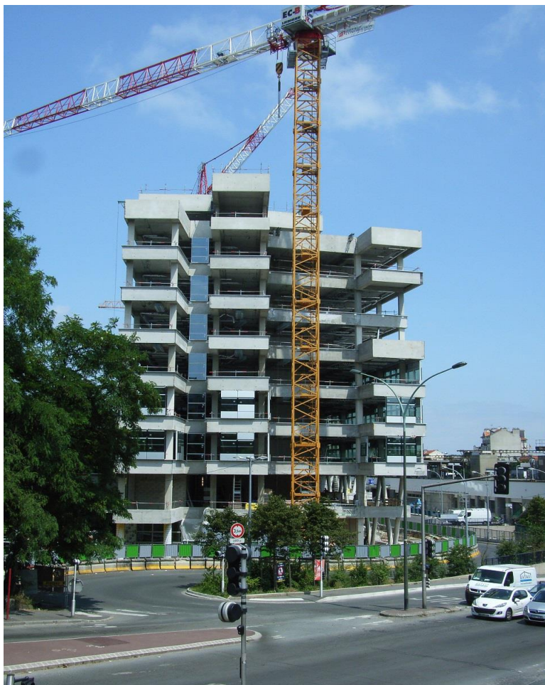
Joinville office development, Paris
