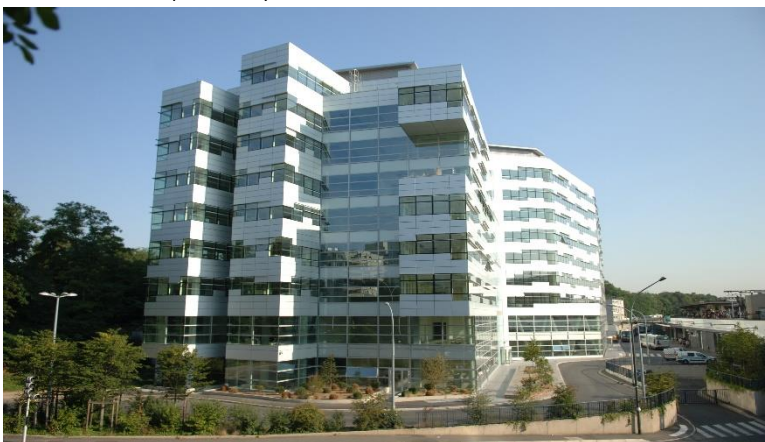
Joinville office development, Paris
