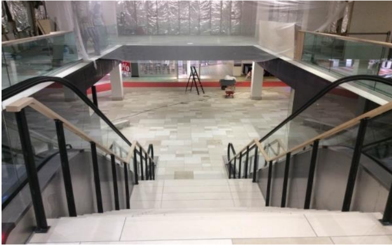
New escalator and floor in Eggert
