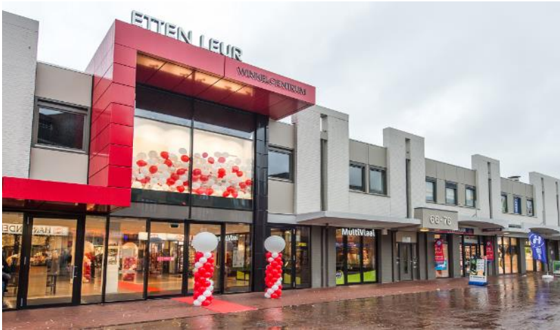
New main entrance in Etten-Leur
