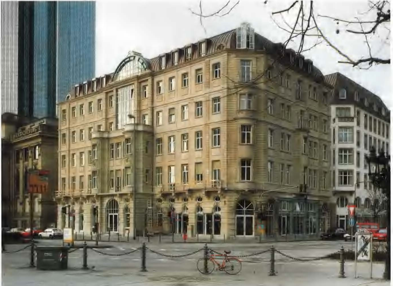
21, Taunusanlage, Frankfurt; refurbished and extended.
