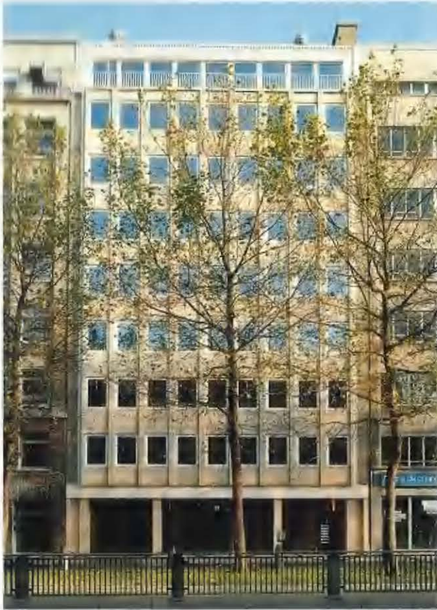
41 Kunstlaan, Brussels, following refurbishment.
