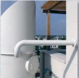
Rainwater storage Rainwater from the roof is stored in large cisterns for irrigation purposes.
