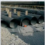
Storm water treatment Underground storm water storage reduces erosion. Rainwater is collected and filtered, and stored in an underground cistern.
