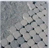
Storm water collection Porous paving is a major element in the management of storm water. Sand and gravel filter the water.
