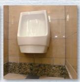
Reduction of water usage Over four billion litres of water are used daily in the US for flushing toilets Waterless urinals and watersaving toilets and shower heads reduce water usage by 50%.
