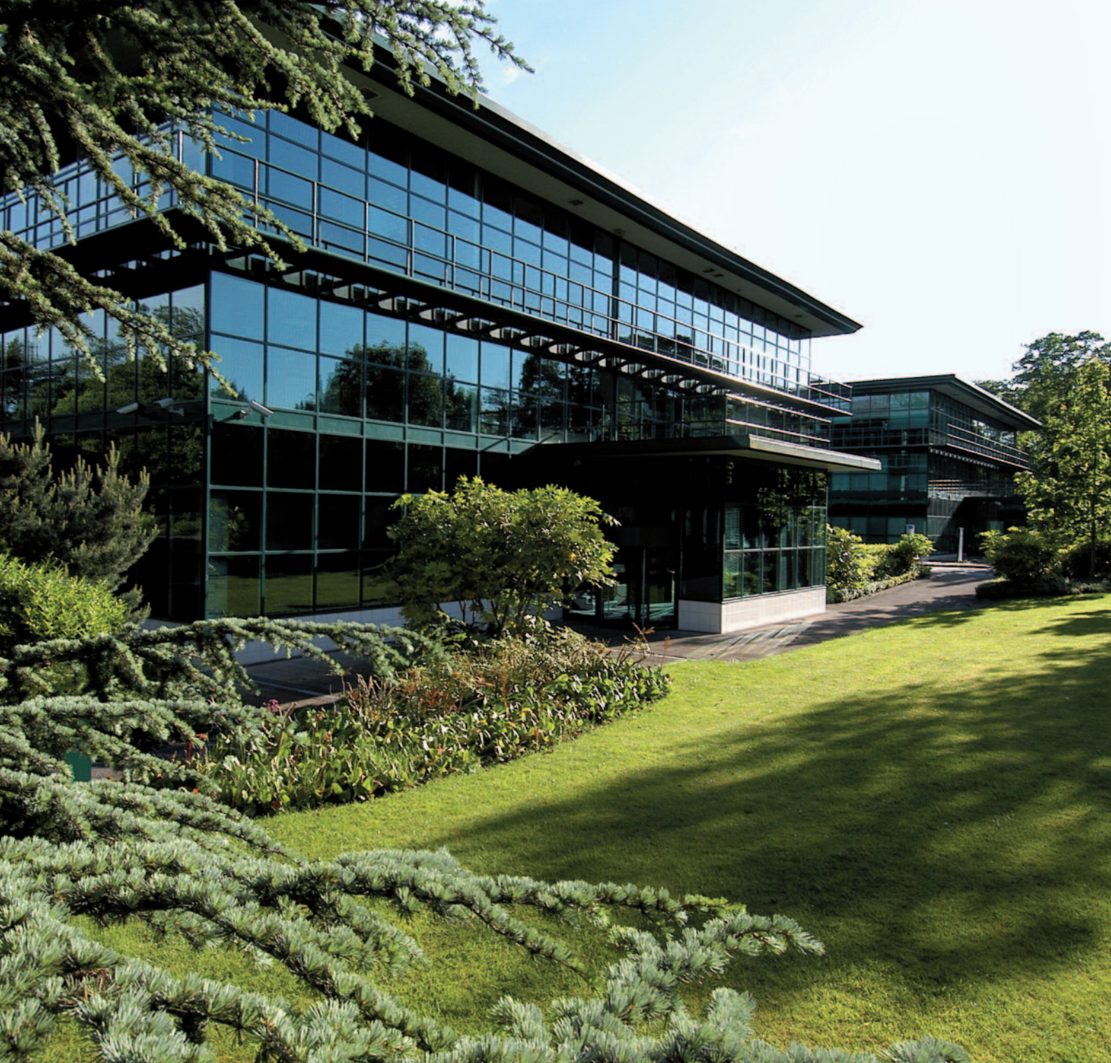
Manchester, The Towers Business Park, Wilmslow Road
