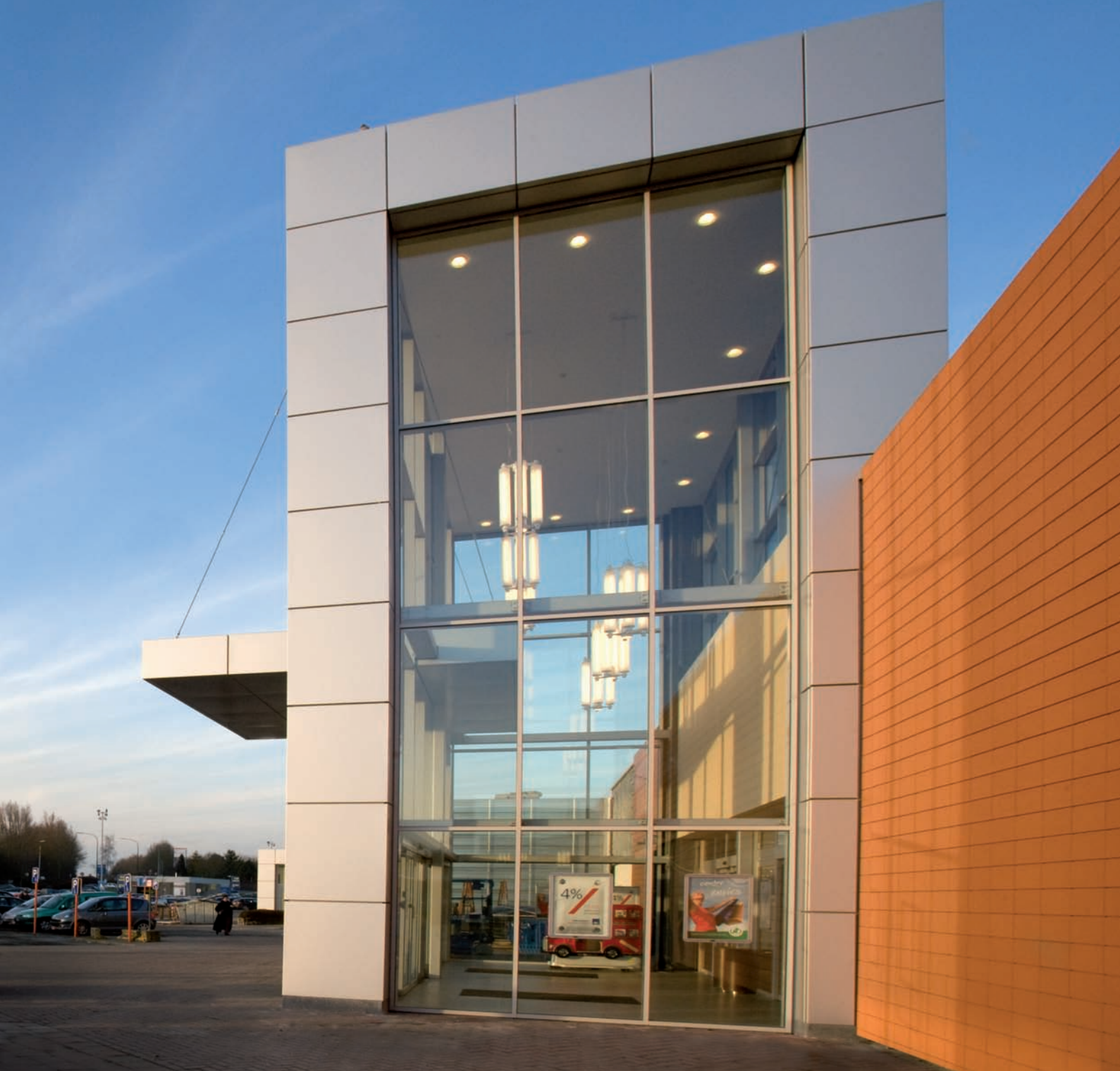
Nivelles shopping centre, Nivelles
